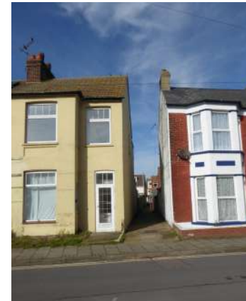
Figure 74 Small spaces between buildings
