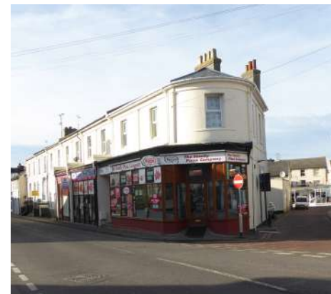
Figure 79 Example of commercial building on corner plot
