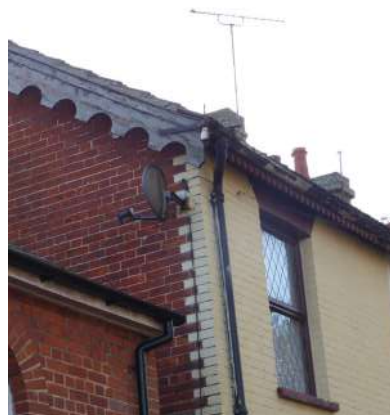
Figure 73 Decorative eaves and corner brick detail
